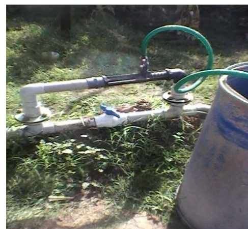
Fig. No. 1: A view of connections of Venturimeter in three acre banana farm
